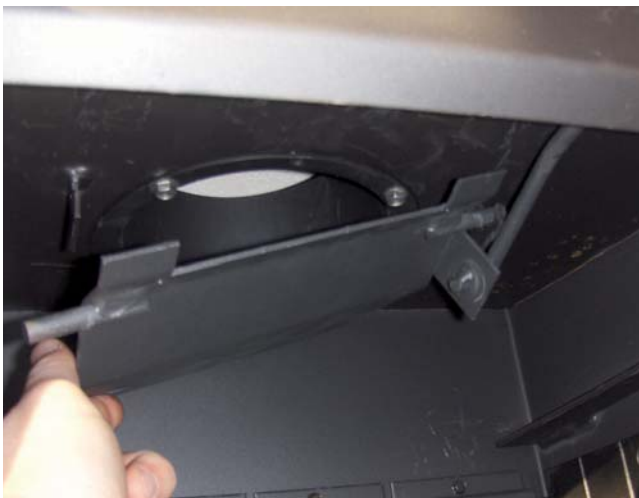
Illustration 1 Remove the pipe collar from the hearth
