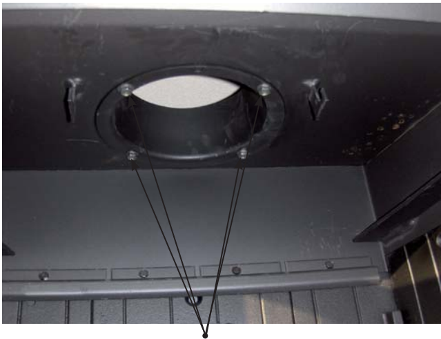
Illustration 1 Remove the pipe collar from the hearth
