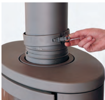
2. Removing the clip bindings from the stovepipe.
